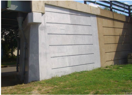
Burlington County, New Jersey, Bridge Abutment Overlook (2017)
