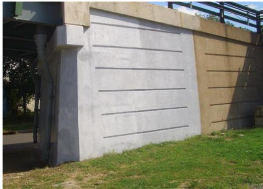
Burlington County, New Jersey, Bridge Abutment Overlook (2017)
